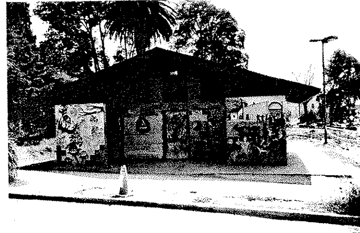
FIGURE 4.7. The front of the restroom and utility building constructed in 1991. It was almost instantly covered with murals and graffiti, much of it depicting the various riots at People's Park and ongoing concerns about police brutality in the city. Photograph by author.
